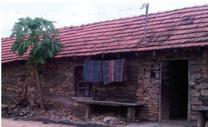
Figure 9: Traditional single-storied dwelling (stone walls, clay-tile roofs).
